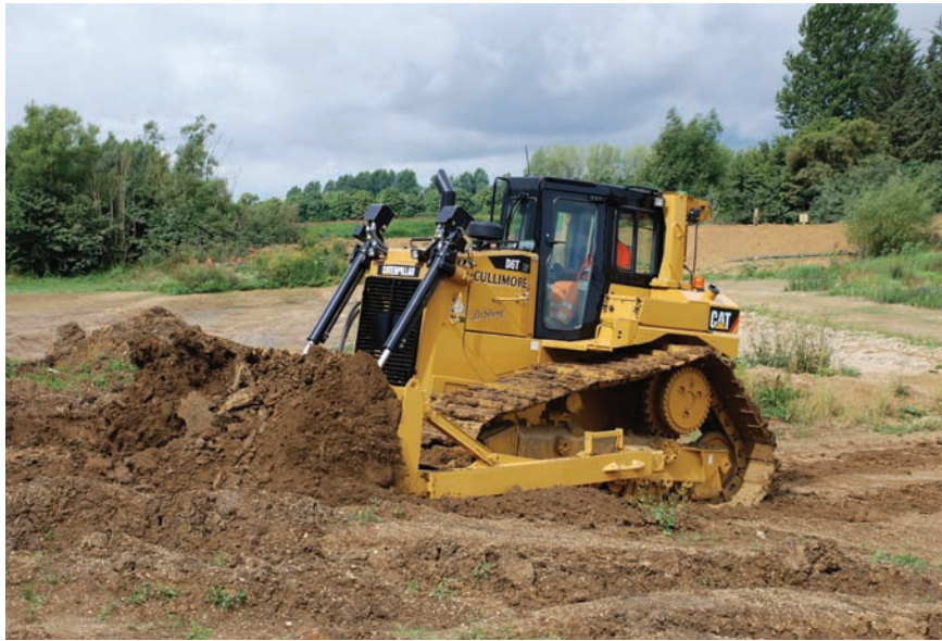
Earthmoving operations at a Cullimore site
