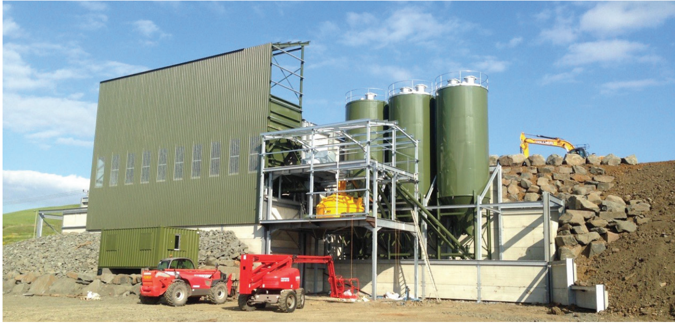
Collier Group's Goathill batching plant under construction
